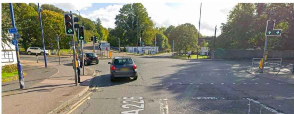
Photograph showing A226 Overy Liberty traffic light junction looking south (to the right) towards Kent Fastway
